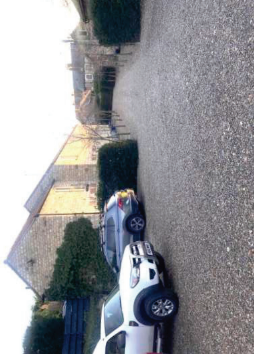
REF PIC D – Looking south east onto the existing Annex accommodation built 2009
