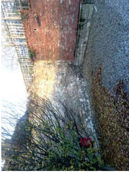
REF PIC E – Looking north east onto 4m retaining wall + fencing
